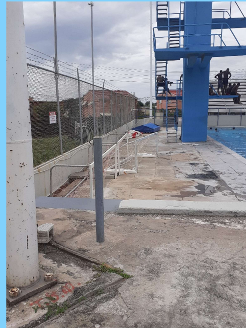
Deck by Diving tower
