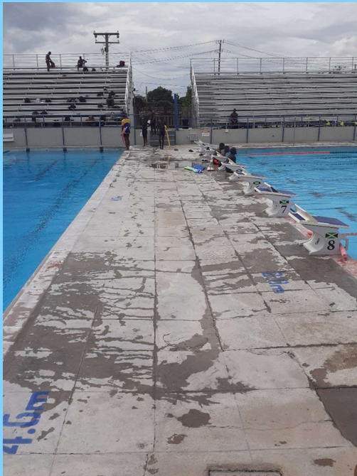
Deck between 25M & 50M Pools
